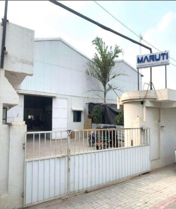
State-of-the-Art and Tech- focused Manufacturing Facility at Veraval (Shapar), Rajkot
